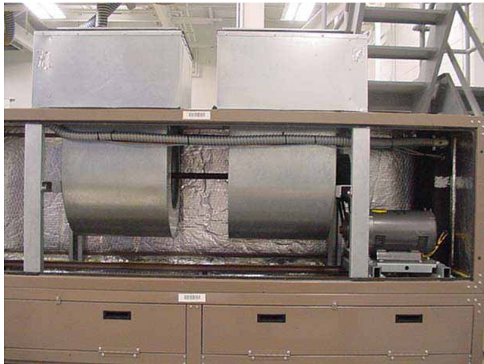
FIGURE 7 - CONDUIT BEHIND BLOWER
